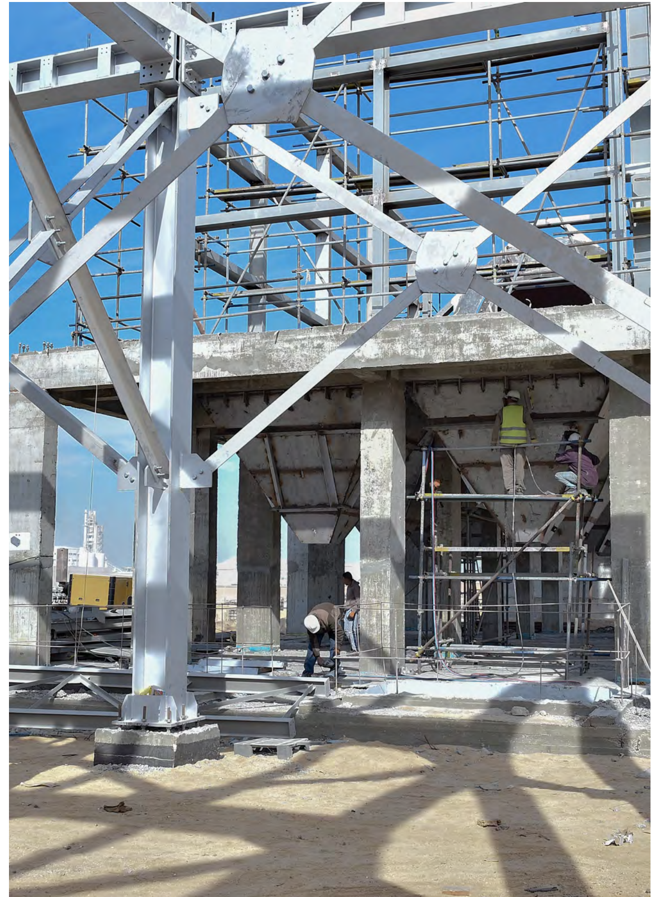
Client: Cyprometal Project: Zinc Smelter Factory GSF Scope: Structural steel, Mechanical work, Plate work, Hoppers, Filters, Silos, Tanks, Conveyors Total Quantity: 3.000 Tonnes
