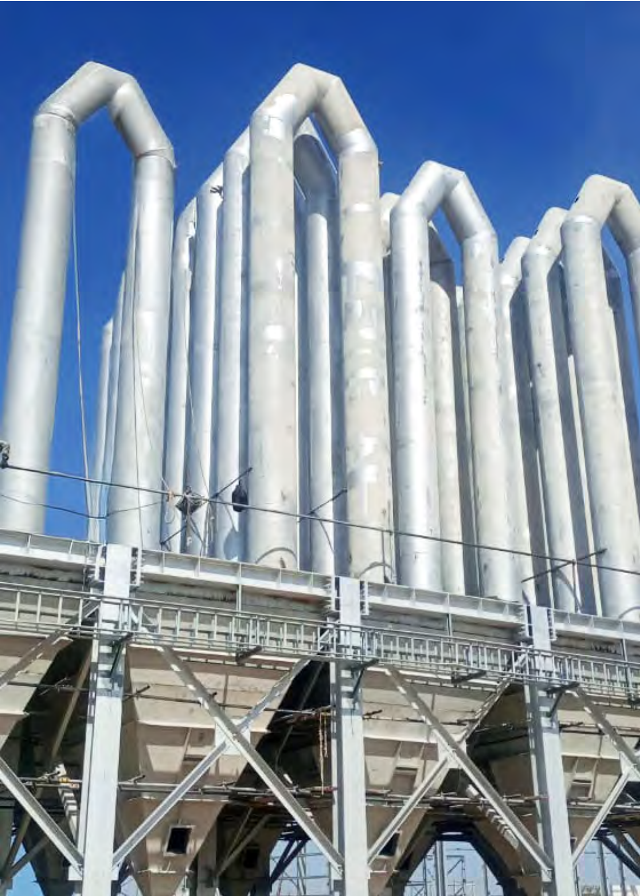
Client: Cyprometal Project: Zinc Smelter Factory GSF Scope: Structural steel, Mechanical work, Plate work, Hoppers, Filters, Silos, Tanks, Conveyors Total Quantity: 3.000 Tonnes
