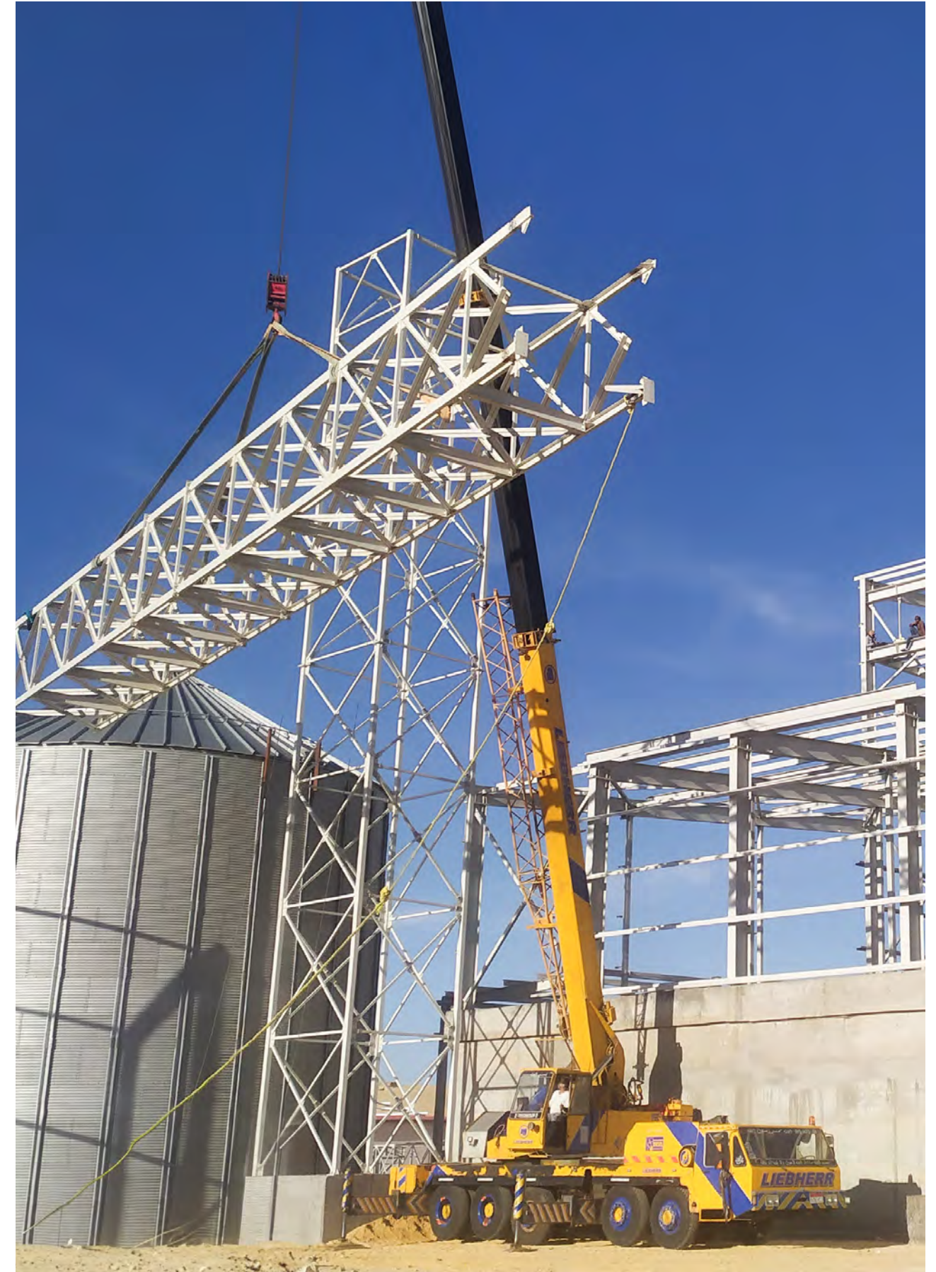
Client: Global Company Project: Chicken Feed Factory GSF Scope: Supply and installation of structural steel Total Quantity: 275 Tonnes
