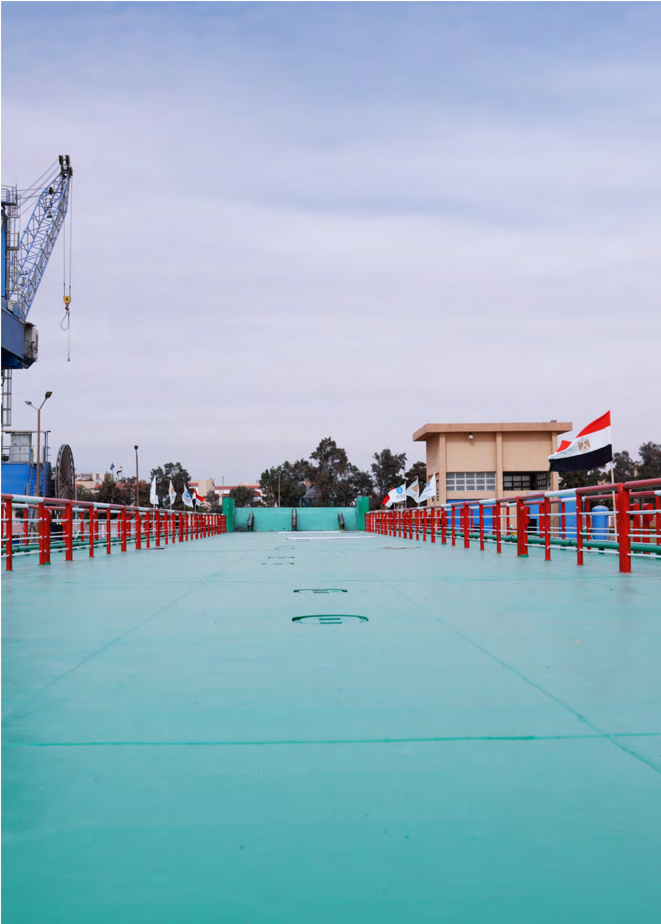
Client: Suez Canal Authority GSF Scope: Fabrication of Marine Pontoons
