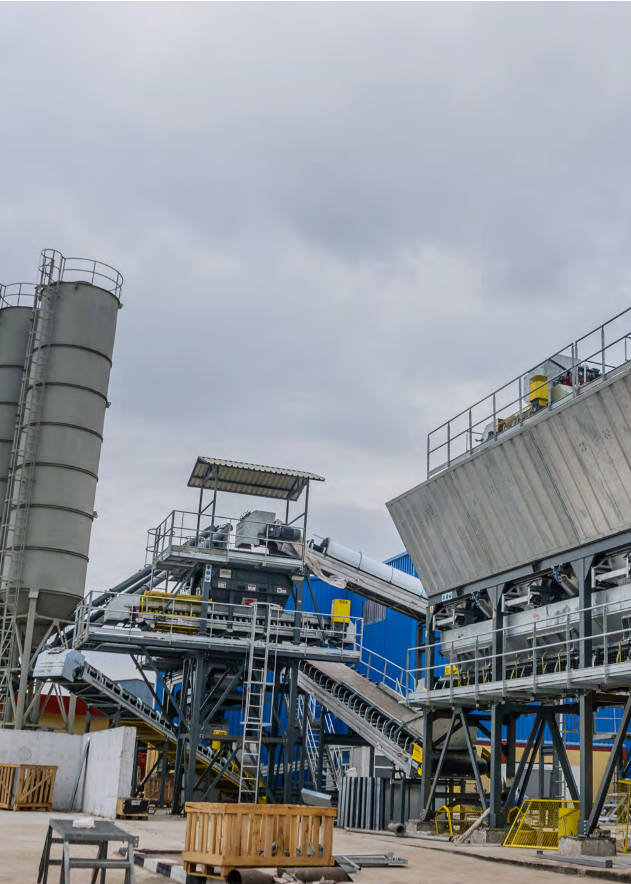
Client: Petrojet Project: Pipes concrete coating factory GSF Scope: Installation of structural steel and mechanical equipment
