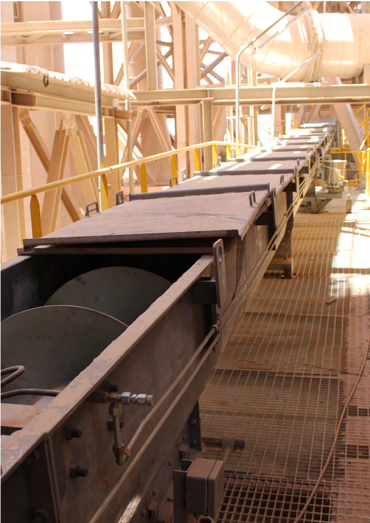
Client: Arabian Cement Company Project: Screw conveyor GSF Scope: Supply and installation of Screw conveyor
