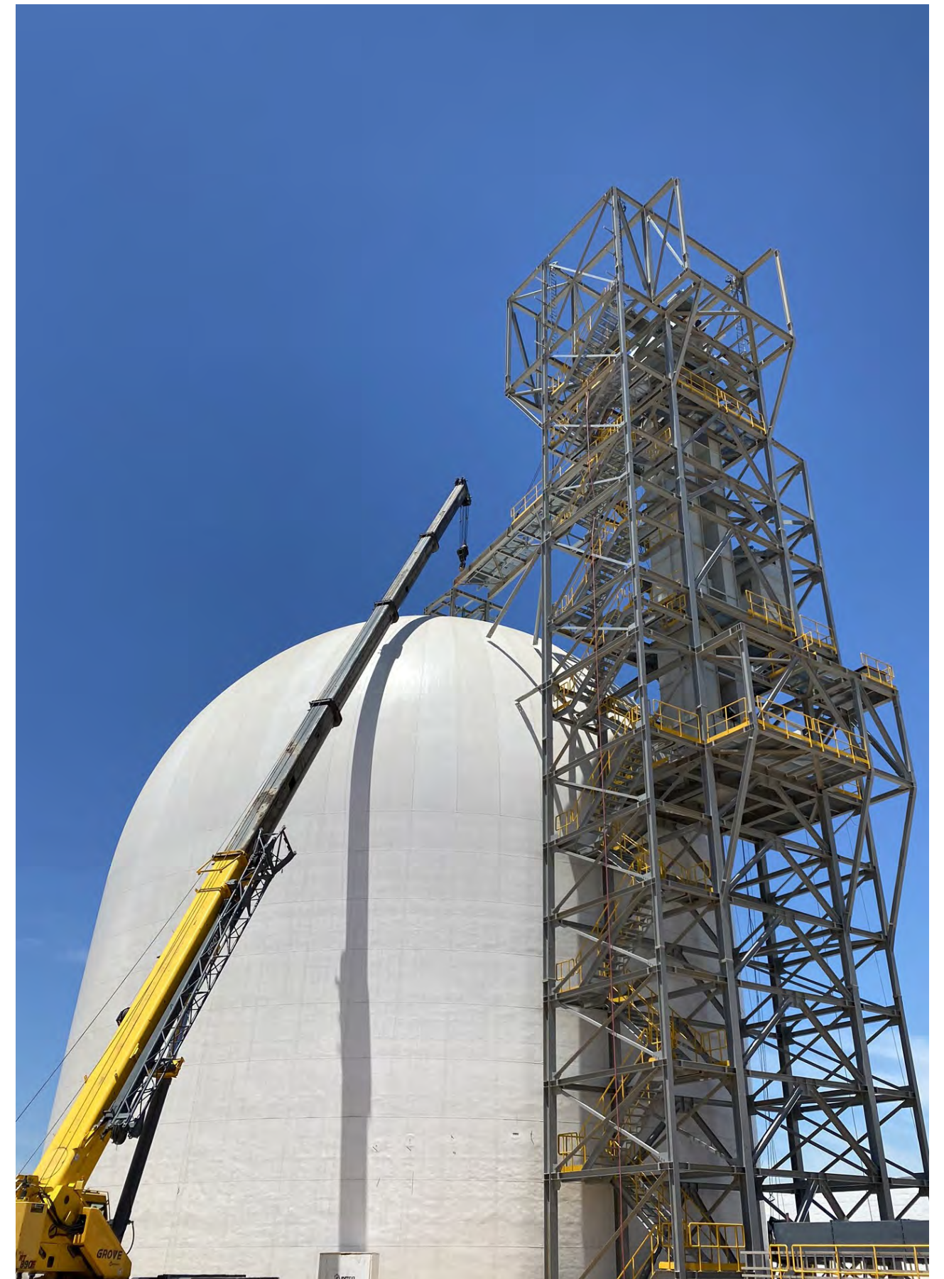
Client: BBM Terminal Corp. Houston, USA Project: BBM terminal GSF Scope: Supply structural steel
