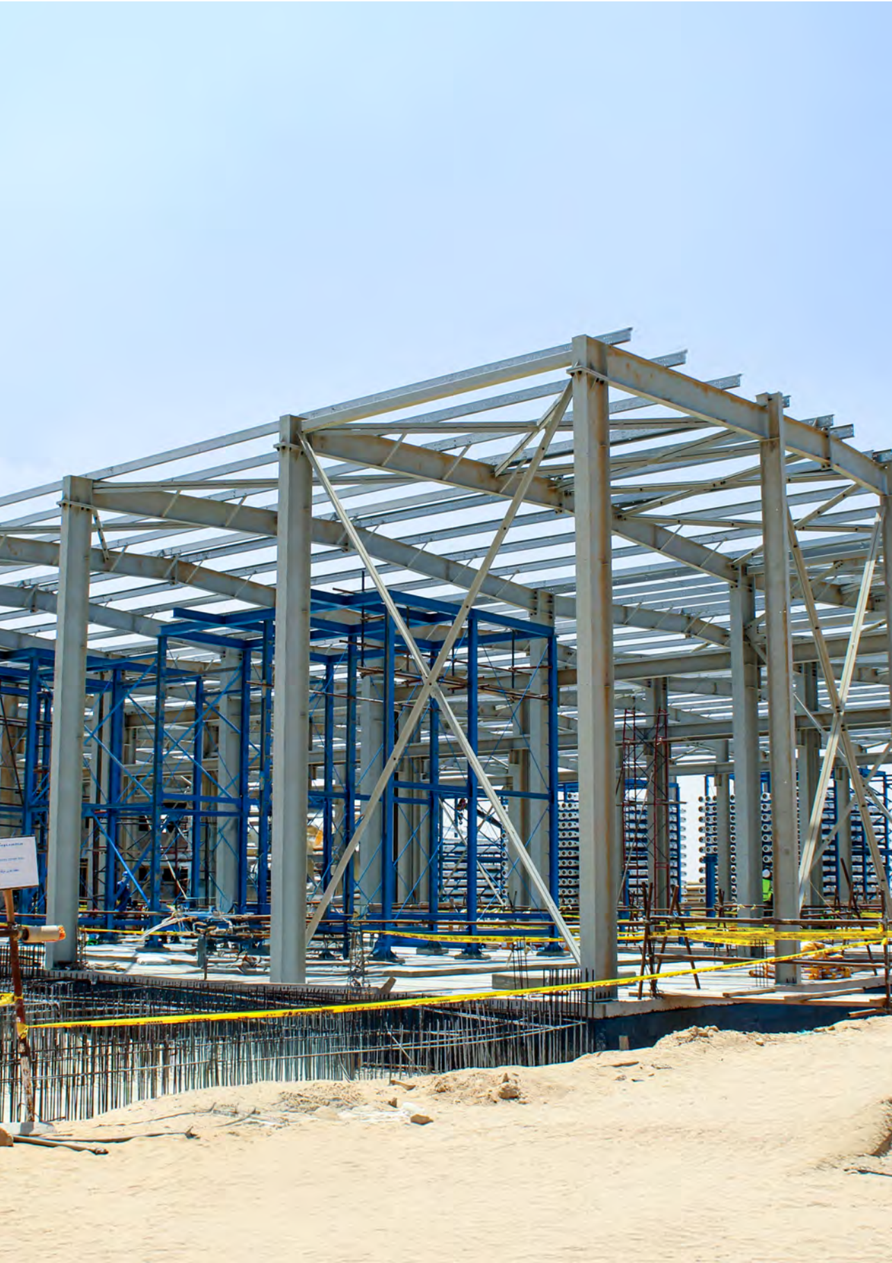
Client: FCC Aqualia Project: Al-Alamen water desalination plant GSF Scope: Supply and installation of structural steel
