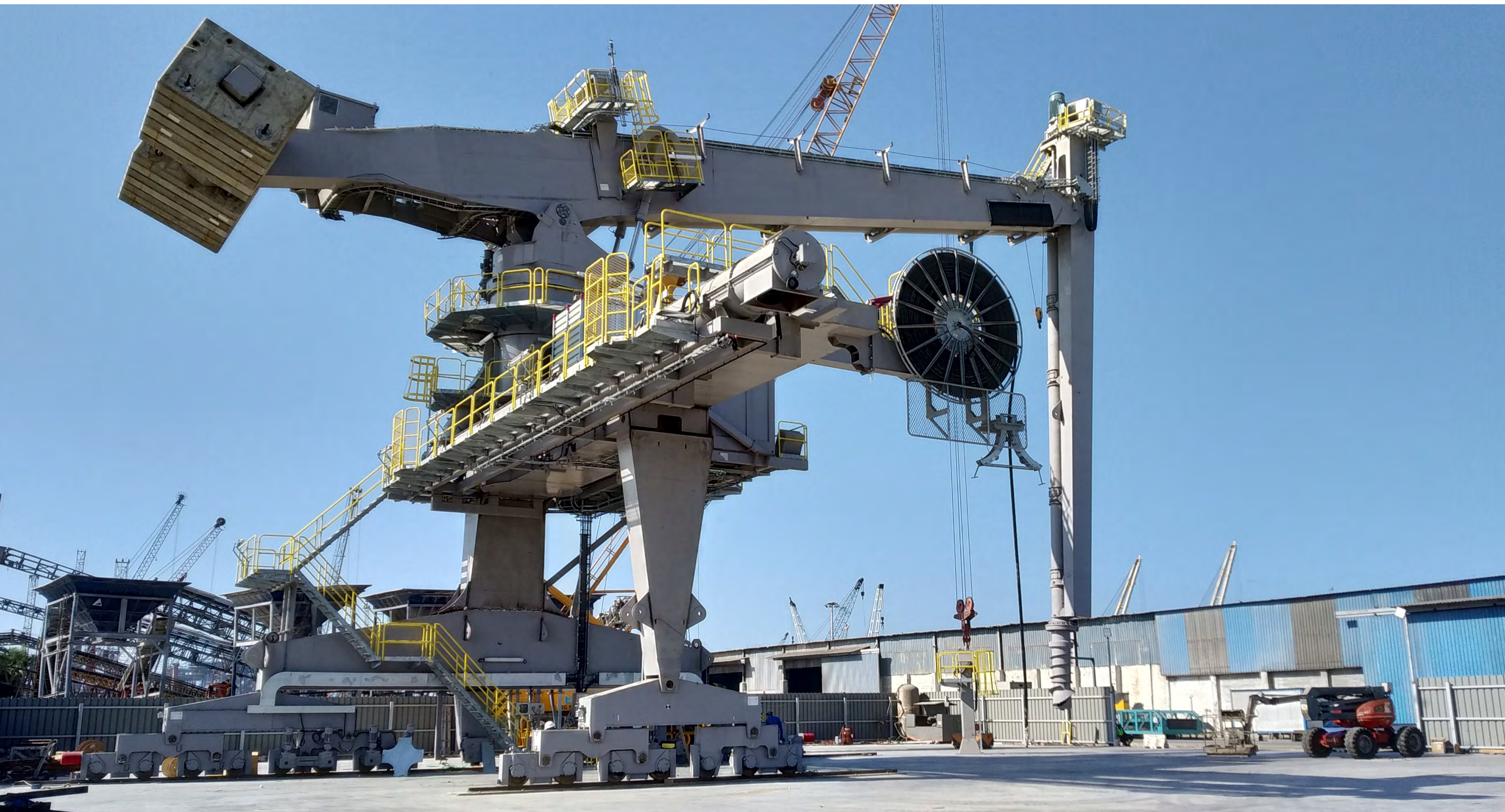
Client: BBM Terminals Corp. - USA Project: Ship unloader GSF Scope: Mechanical & Electrical
