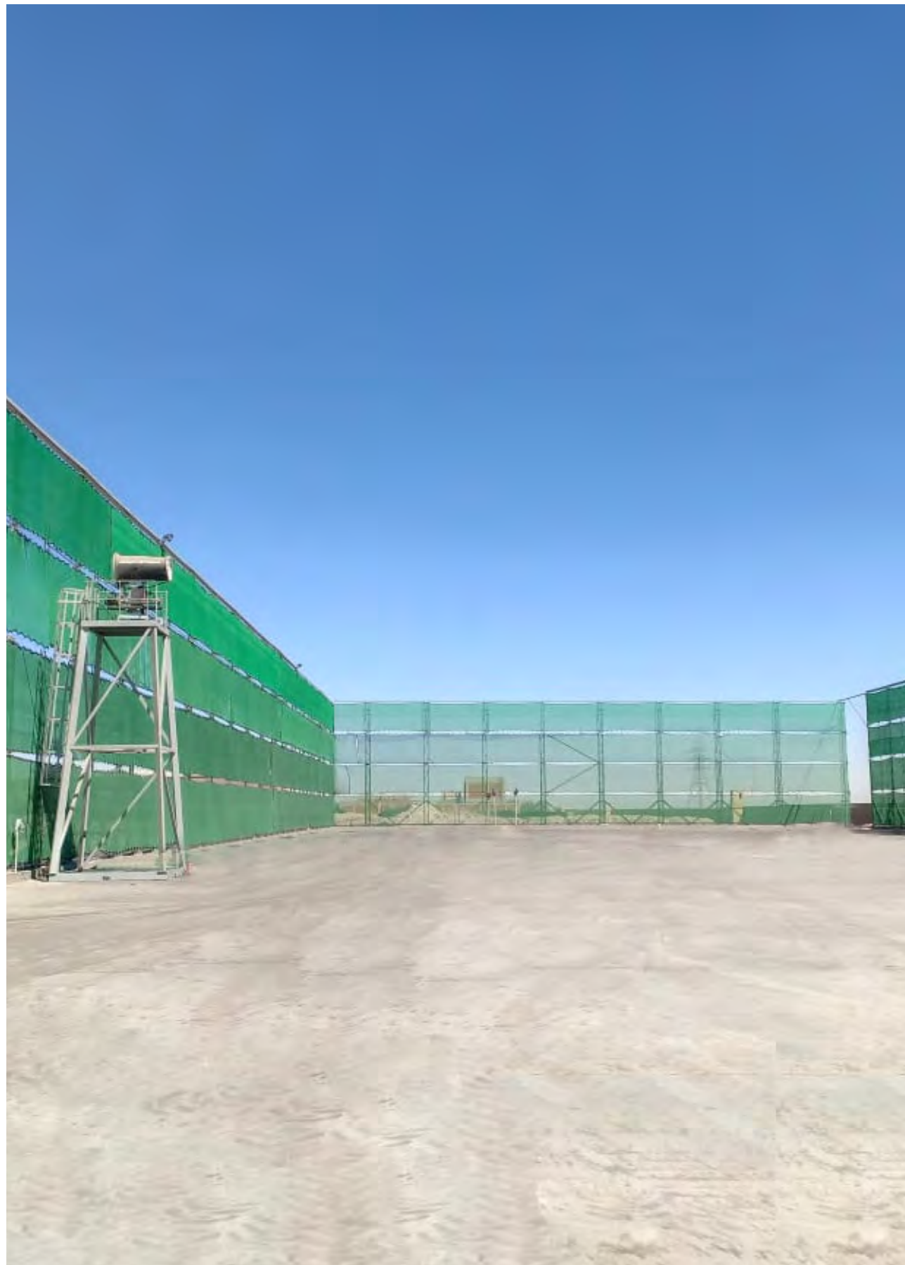
Client: BMIC Project: Coal storage - wind breaker GSF Scope: Turn-Key basis
