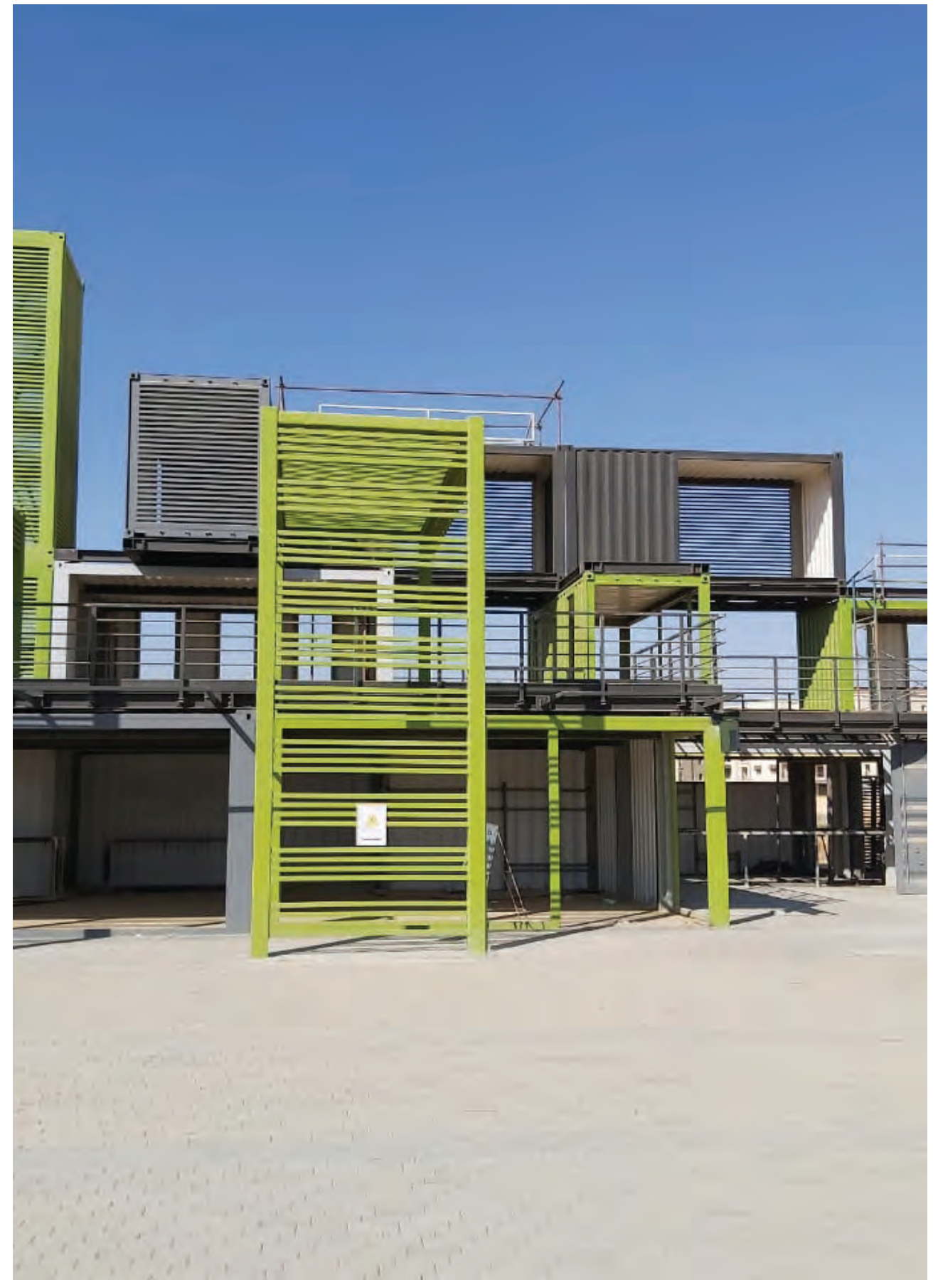
Client: CRC Dorra Project: Mivida Lake District GSF Scope: Supply and installation of Commercial Containers
