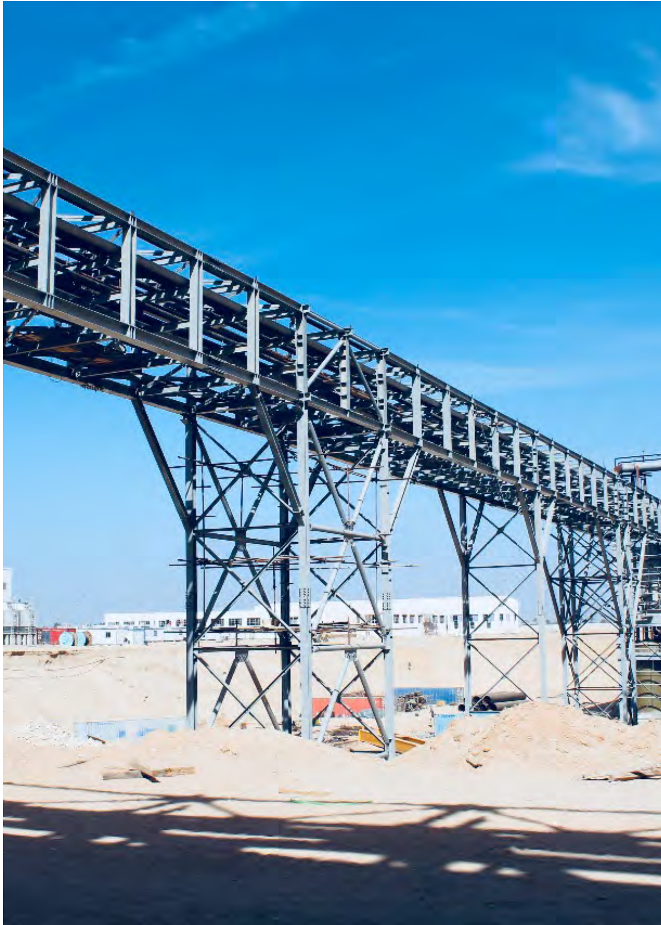
Client: Al Sharkiya Sugar Manufacturing Project: Al-Salhya Factory GSF Scope: Supply and Installation of pipe racks
