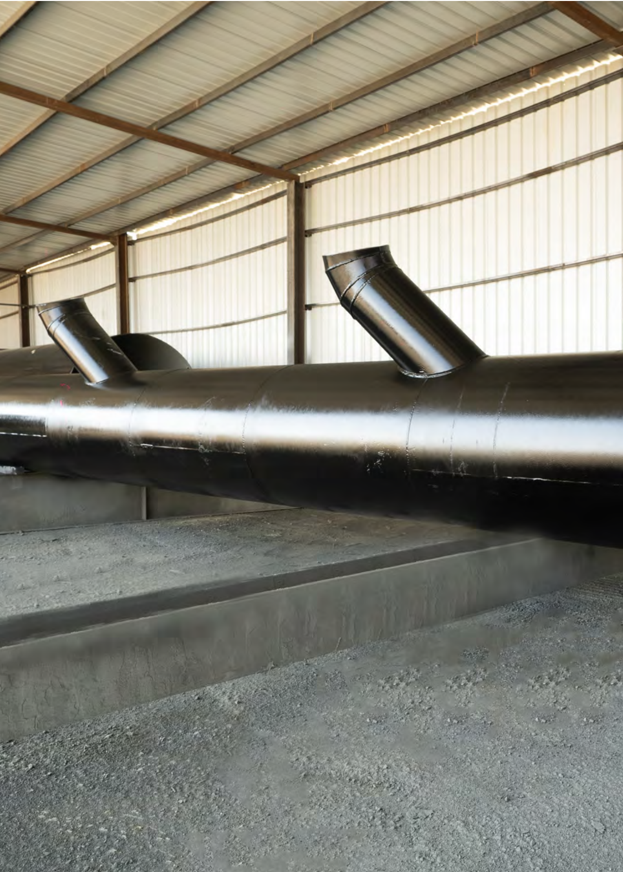
Client: Madkour | Zone: R - TOSHA 35 booster pump stations: Total Length 8,244 m 2 main lifting stations: Total Length 2,000 m Supply & fabrication of carbon steel pipes, fabrication and welding of piping spools, painting of finished pipings
