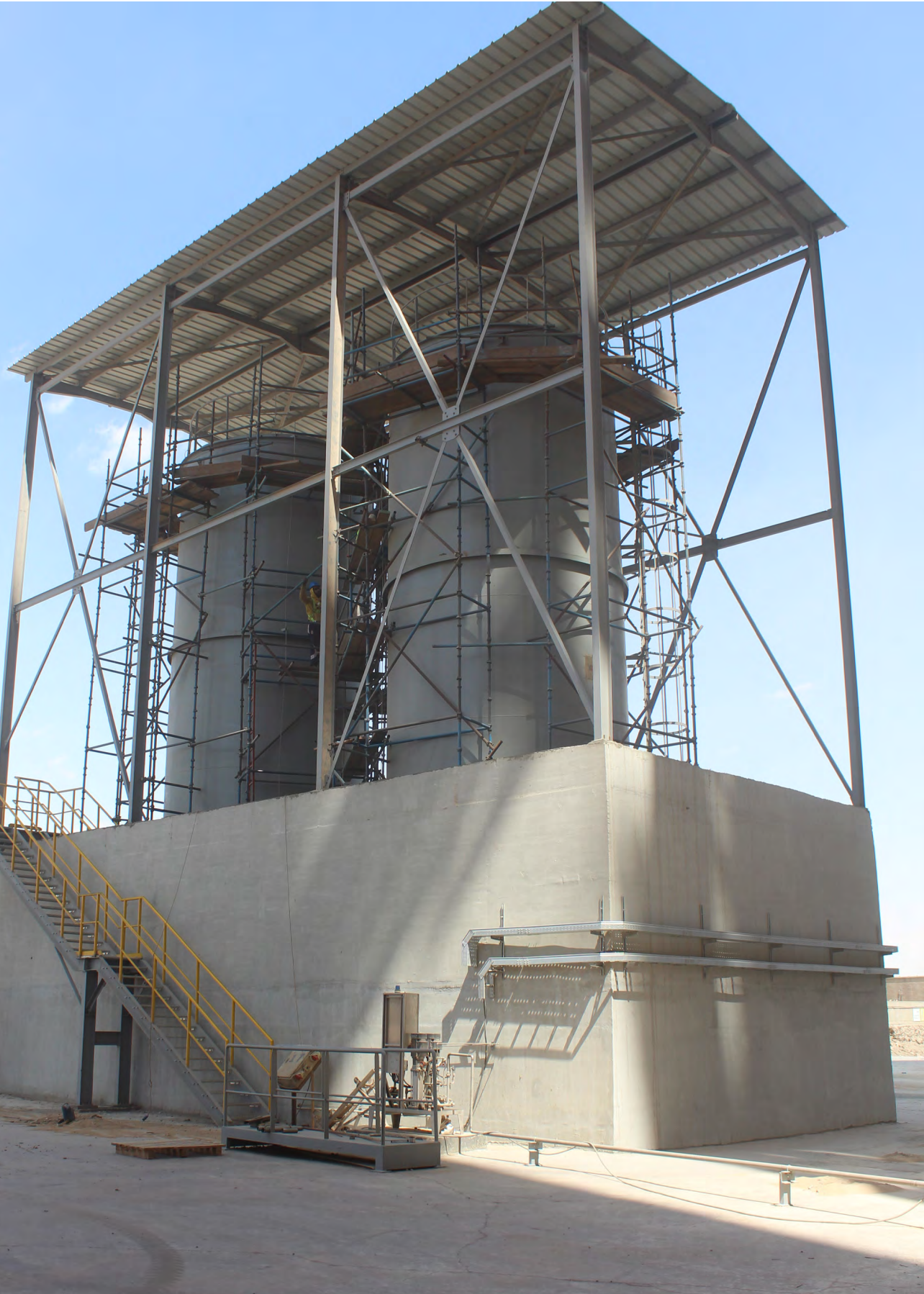
Client: Arabian Cement Company Project: Double wall ammonia tanks GSF Scope: Design, fabrication, supply, installation, test & commissioning of two double wall
