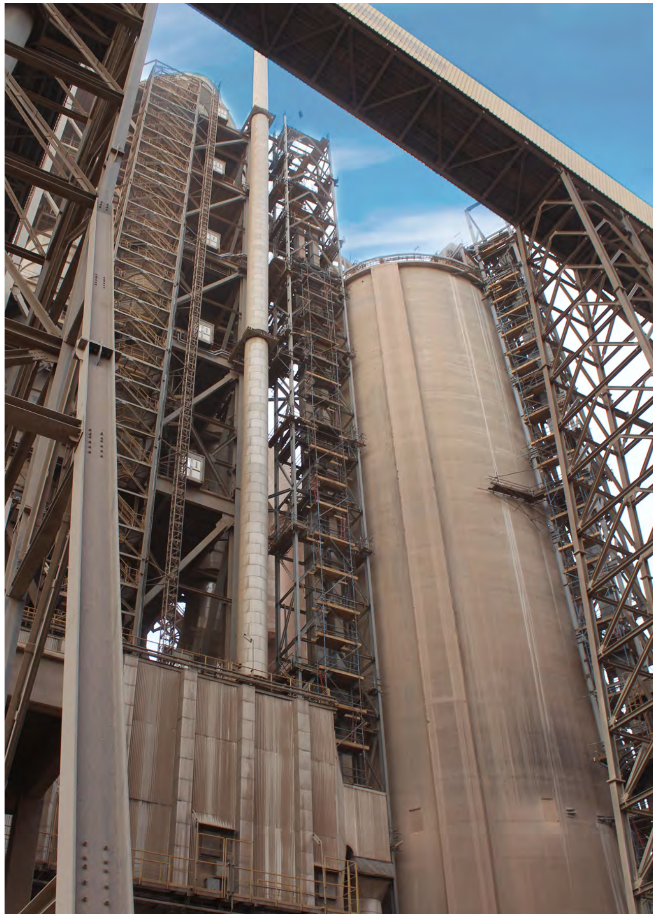
Client: Arabian Cement Company Project: 2 bucket elevators, Air Slides and Screw Conveyors GSF Scope: Fabrication, supply and installation
