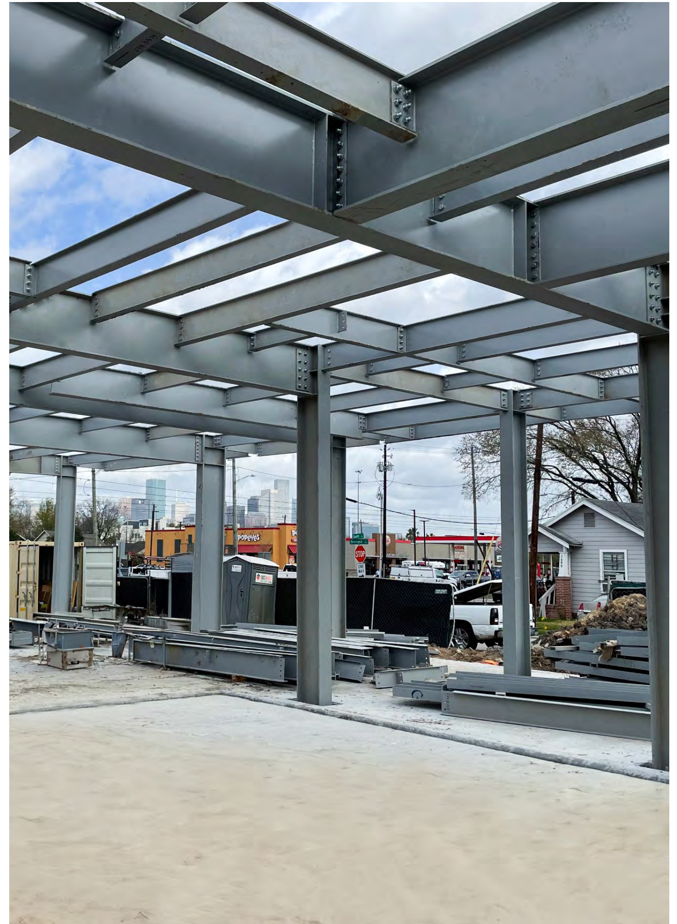
Client: CIVE Project: Students Housing podium structure GSF Scope: Supply of structural steel Total Quantity: 228 Tonnes
