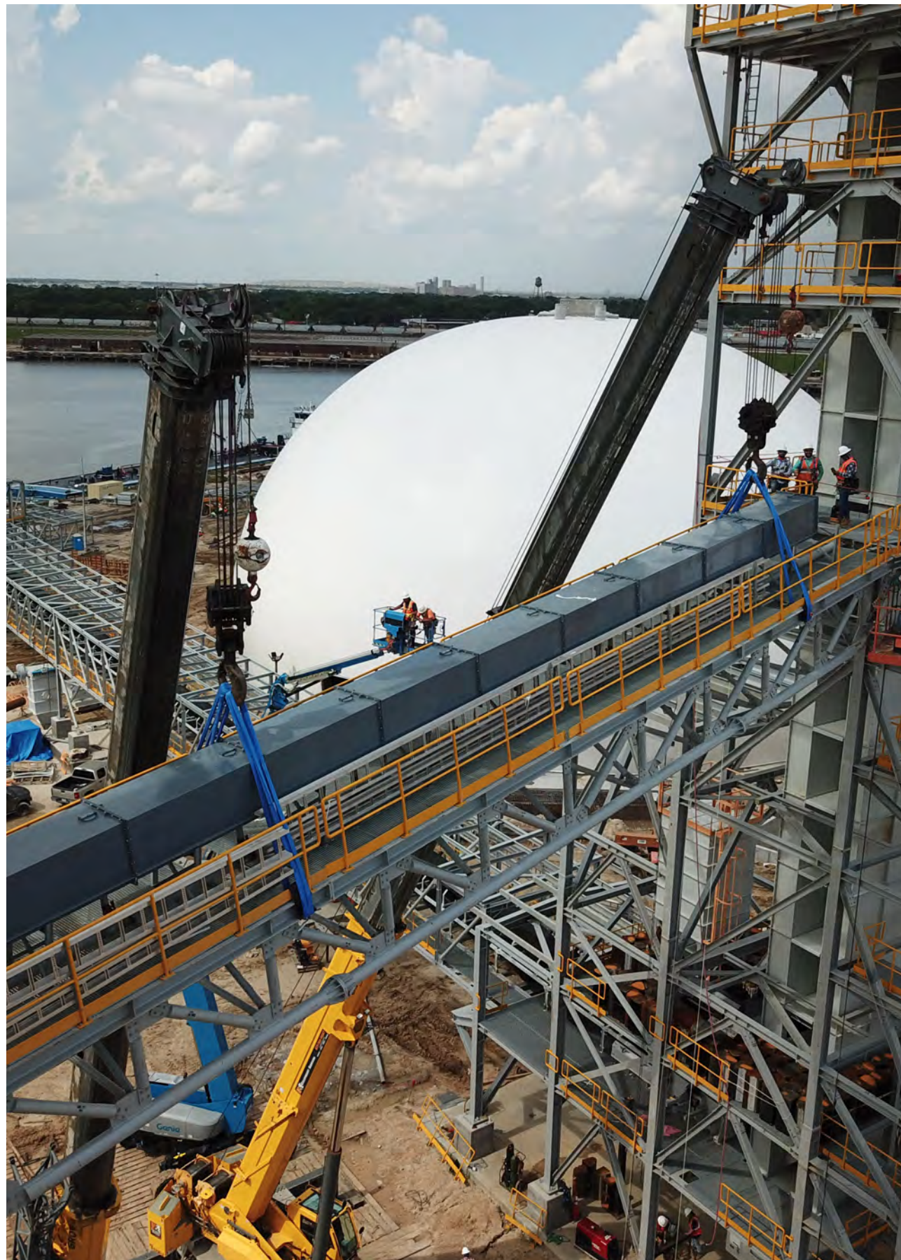
Client: BBM Terminal Corp. Houston, USA Project: BBM terminal GSF Scope: Supply structural steel
