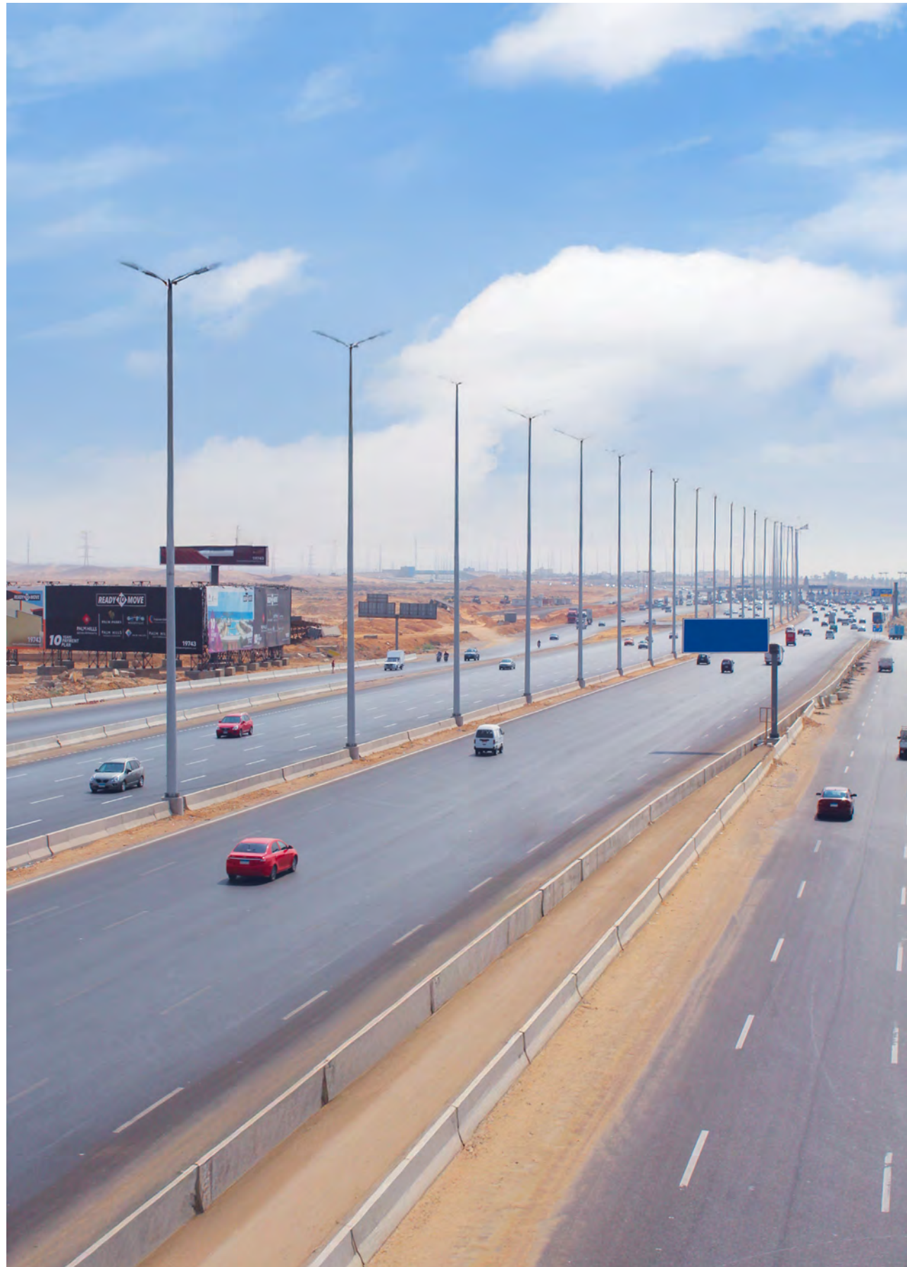
Client: Elsewedy Electric Project: Mohamed Bin Zayed Road GSF Scope: Lighting Poles
