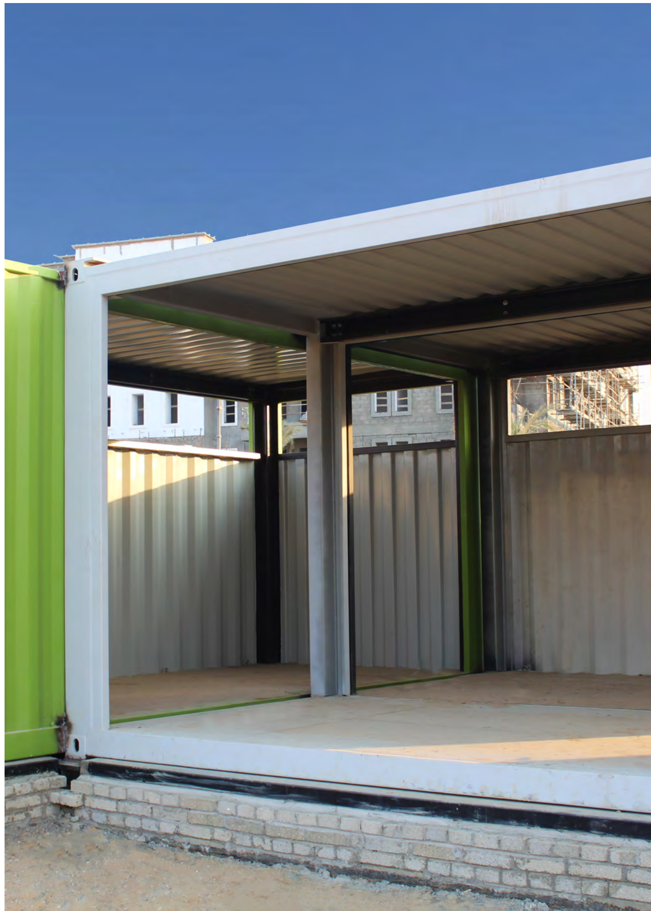
Client: CRC Dorra Project: Mivida Lake District GSF Scope: Supply and installation of Commercial Containers
